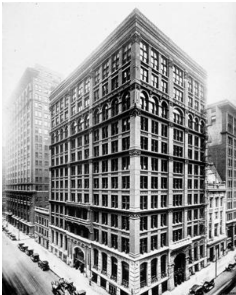
Home Insurance Building Chicago 1885
